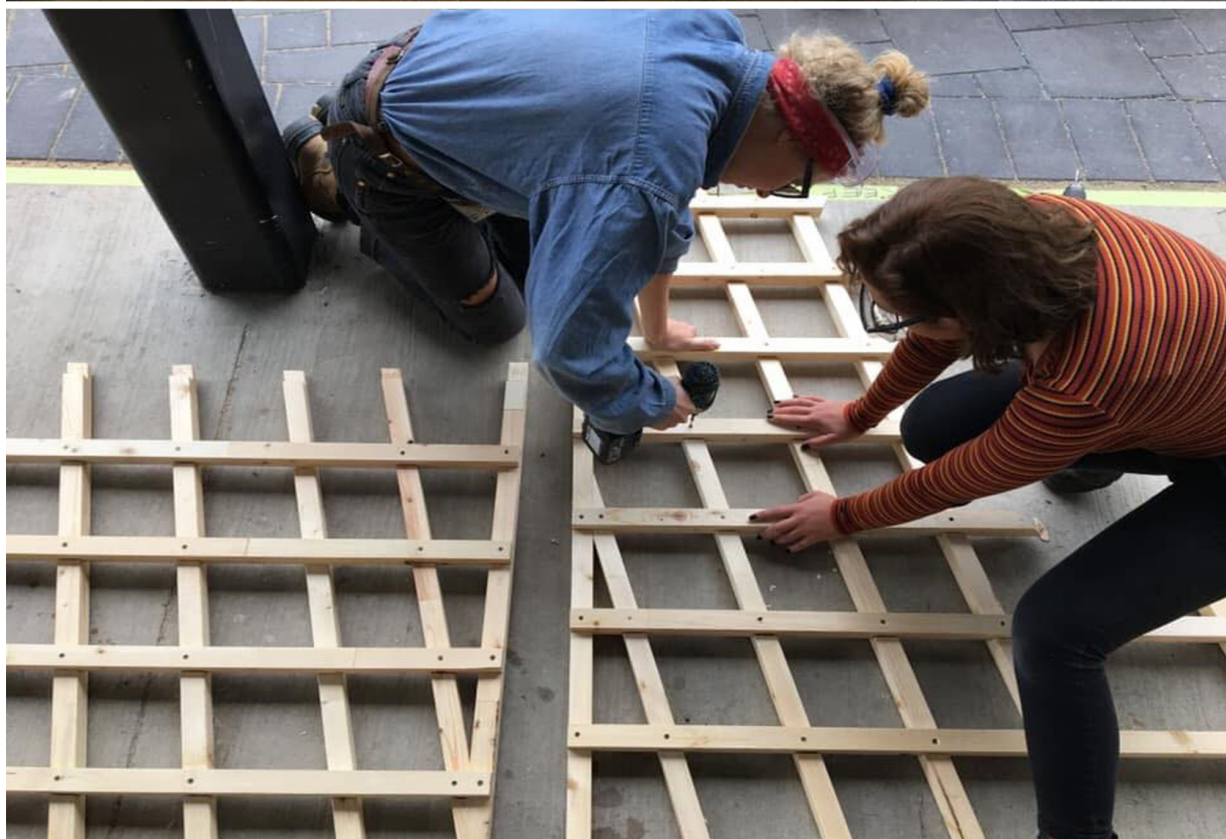
Figure 2. Student fabrication and assembly (Playhouse 2). Image credit: MSOA.
